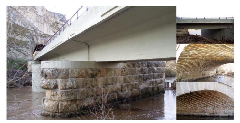
The interventions which took place have been on one hand the construction of a cantilevered service lane on the side of the bridge and on the other the operations of cleaning and structural rehabilitation.
